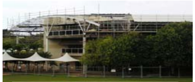
Rust rectification, Level 3, Casuarina Campus
